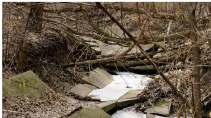
The broken flume will be removed. An underground pipe will be installed and the area will be restored. Photo: UW Arboretum
