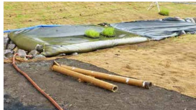
A silt bag will be used to drain Curtis Pond. The permeable material will collect sediment as water flows through it. Photo: Strand Associates
